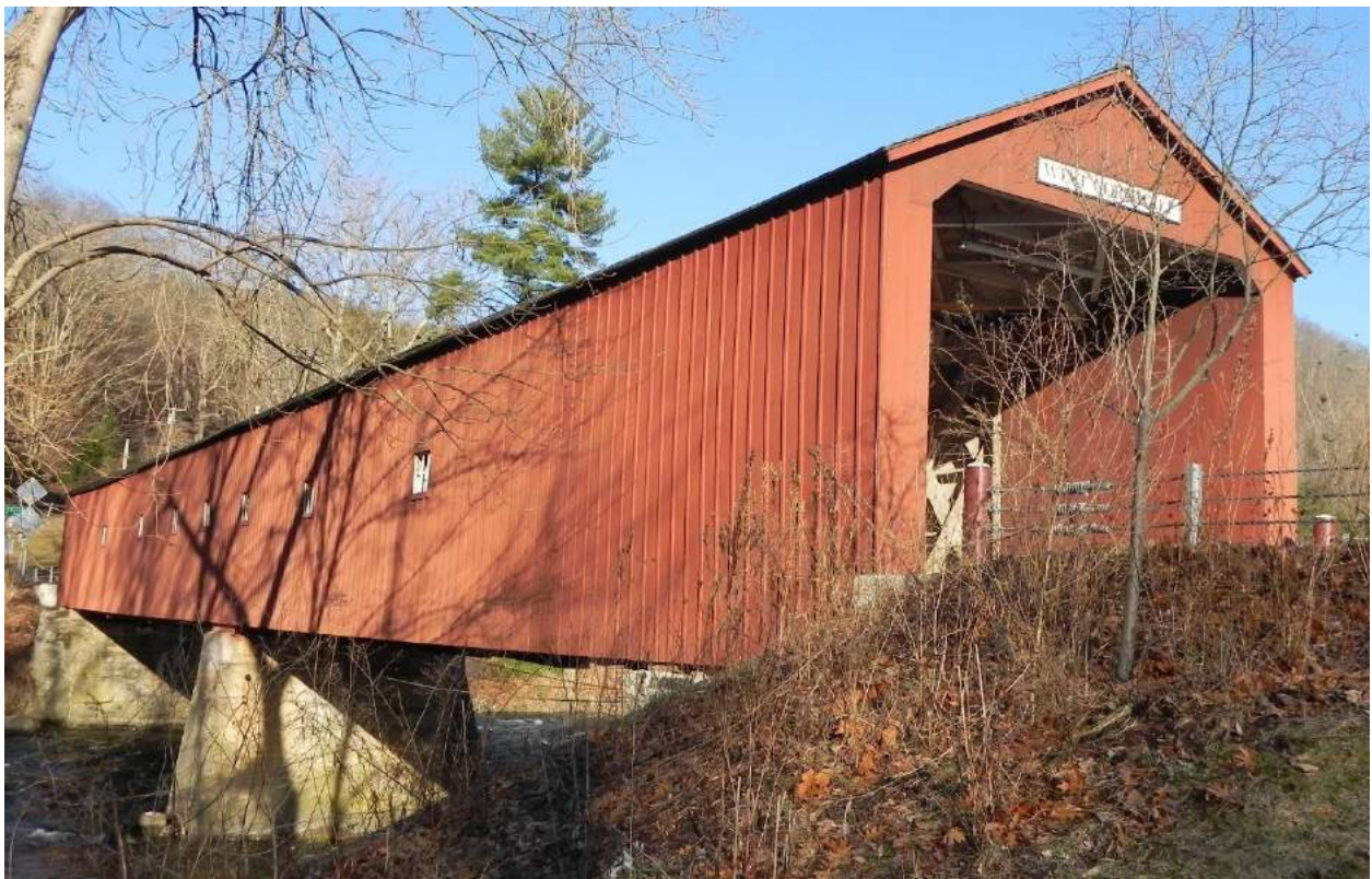
West Cornwall bridge
