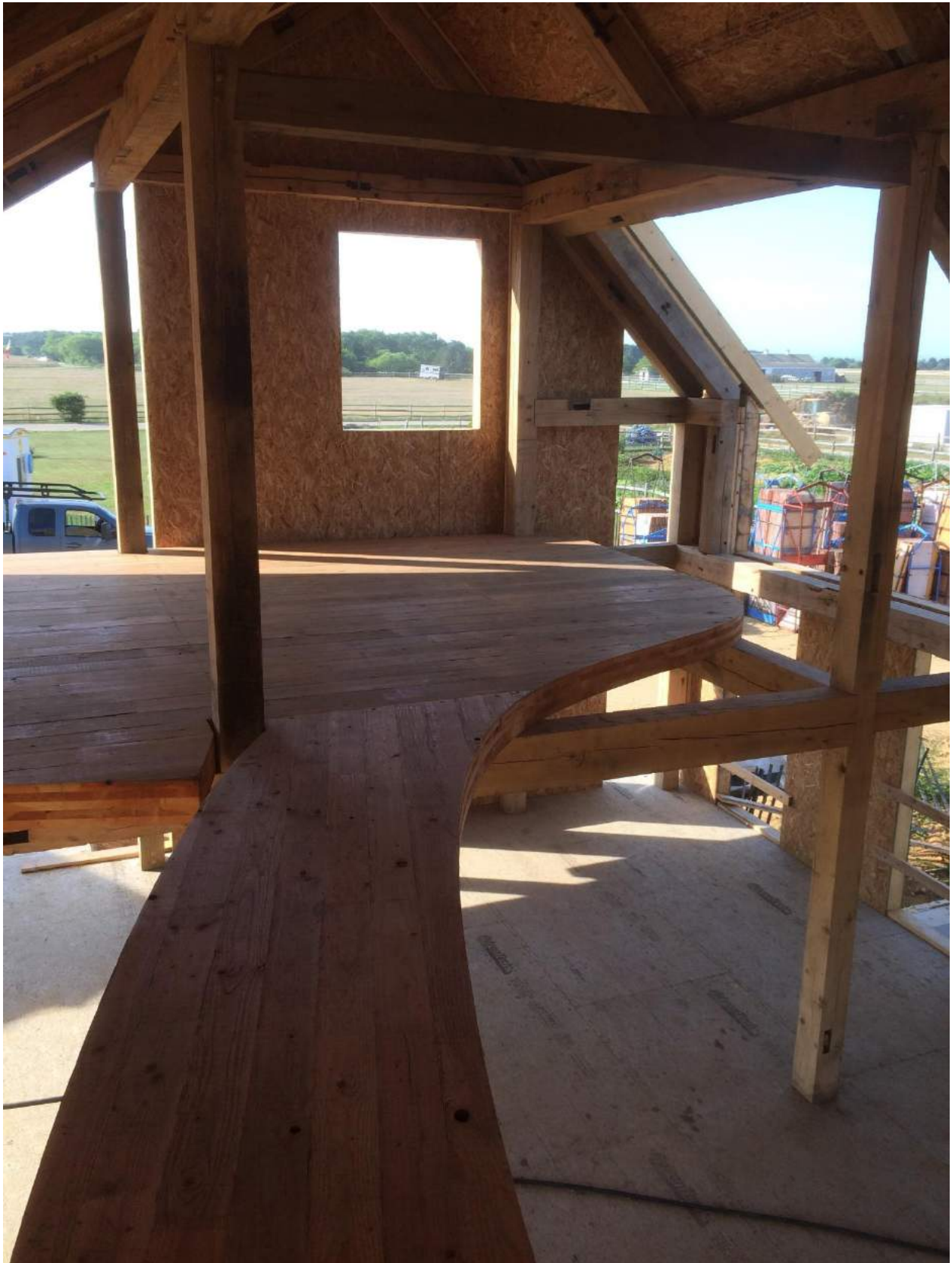
CLT floor panels with curvilinear shapes
