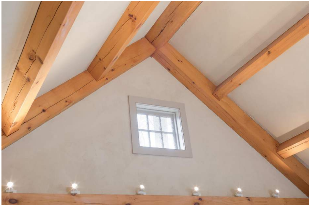
Light fixtures mounted on top of the timbers bounce light off a plaster ceiling; photo credit – Tim Lee Photography
