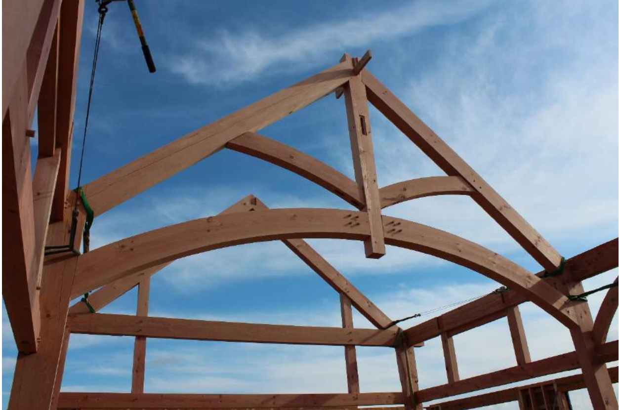
Grain matched curved truss bottom chord
