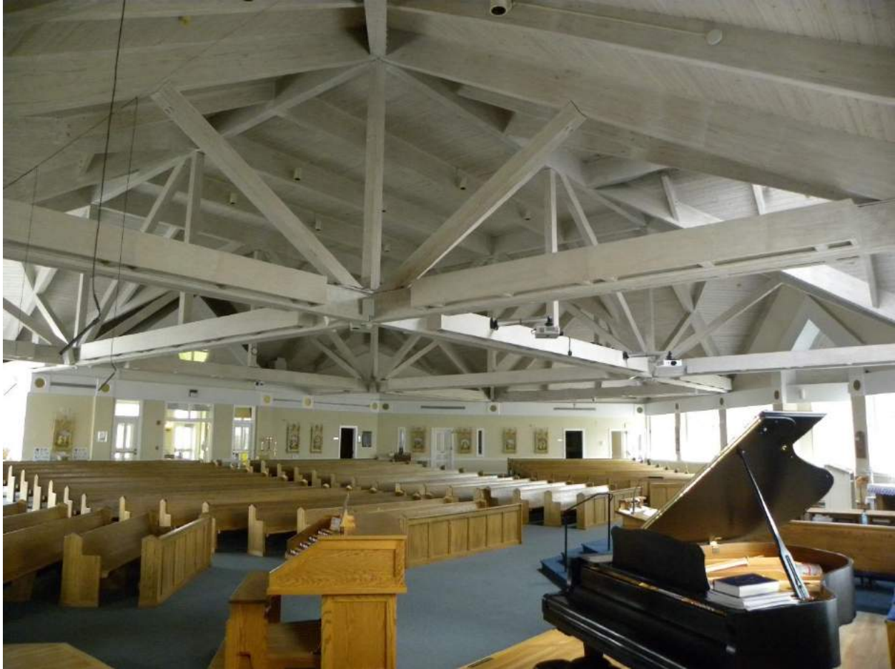
Glulam timber structure with nearly invisible connections
