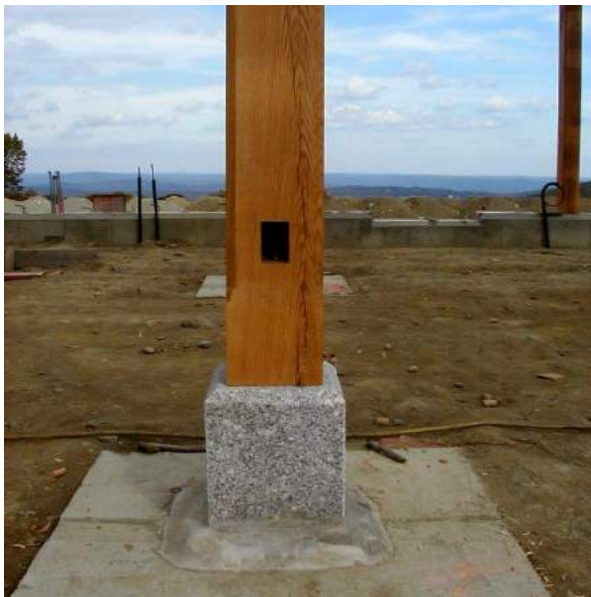
Granite plinth keeps the timber post base high and dry
