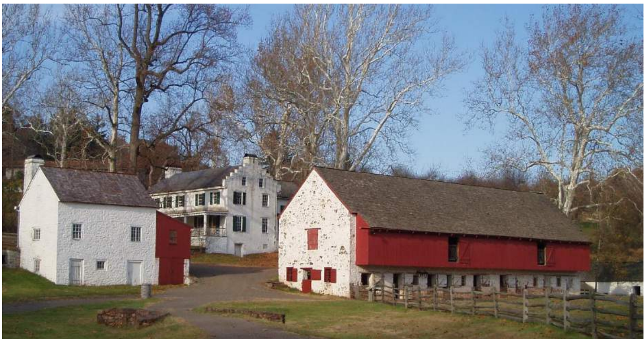
Pennsylvania barn with stone end walls
