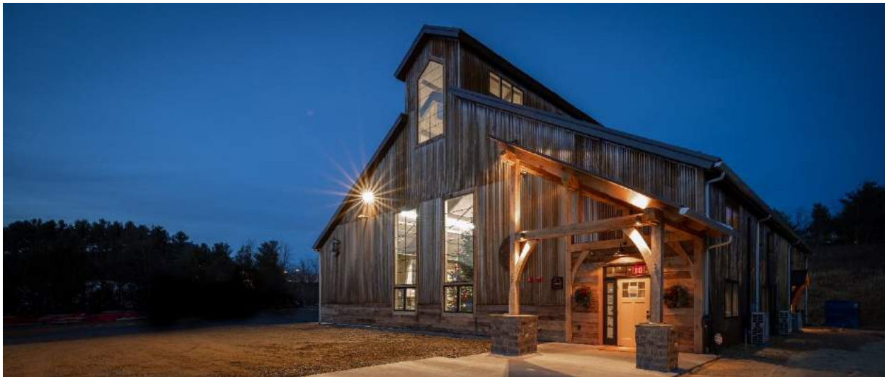
State of the art timber shop in West Jefferson, NC
