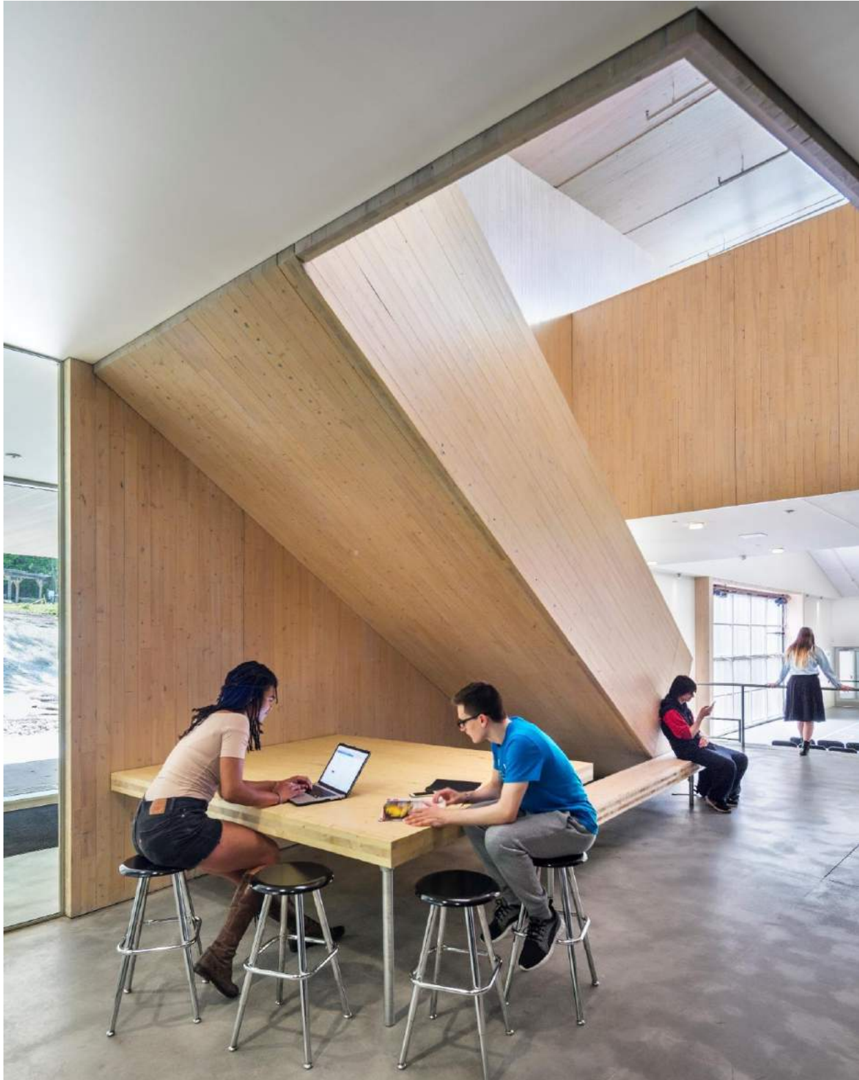
CLT panels were used for the entire structure and everything else, including stairs, tables, and benches at the Common Ground High School designed by Gray Organschi Architects. photo credit – David Sunderland / Esto
