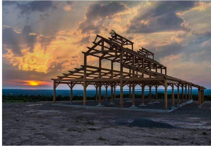
Timber sunrise; photo credit – New Energy Works
