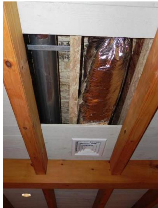
False floor provides a space for utilities
