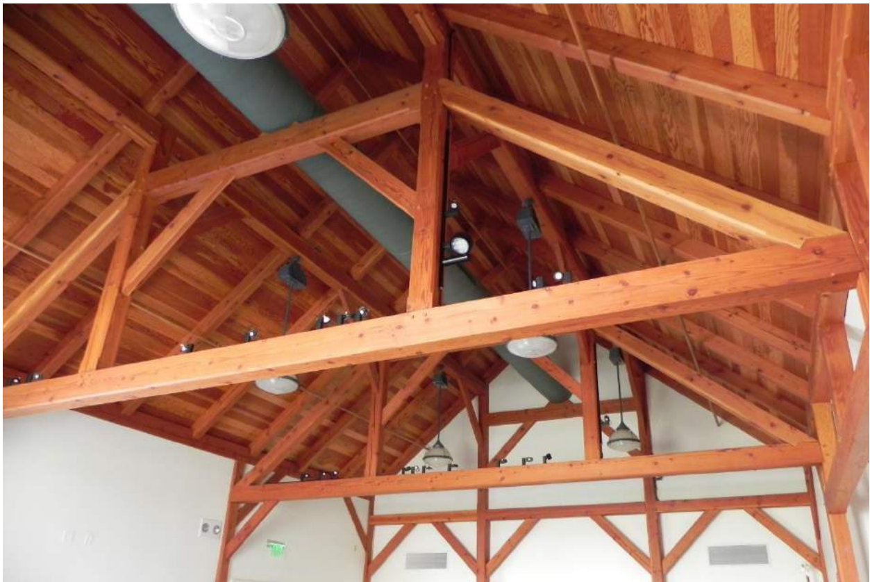
Douglas Fir queen post trusses
