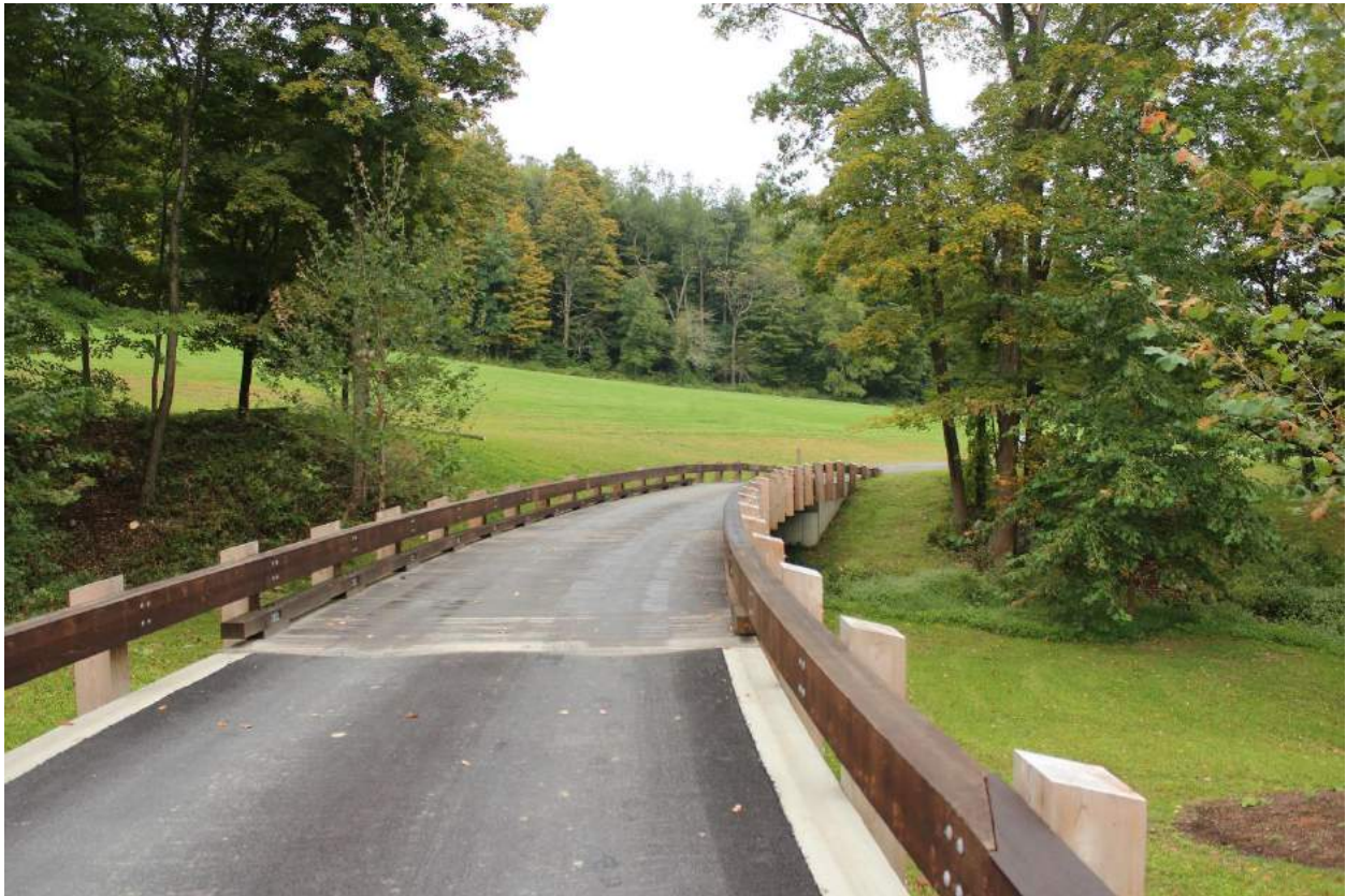
Country lane bridge
