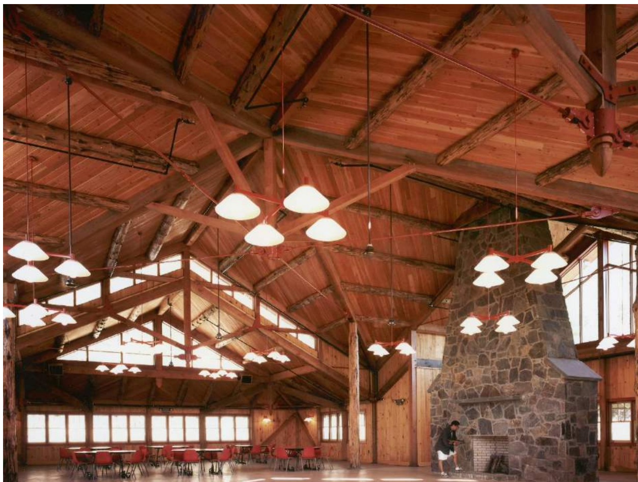
Timber framing – Vermont Timberworks
