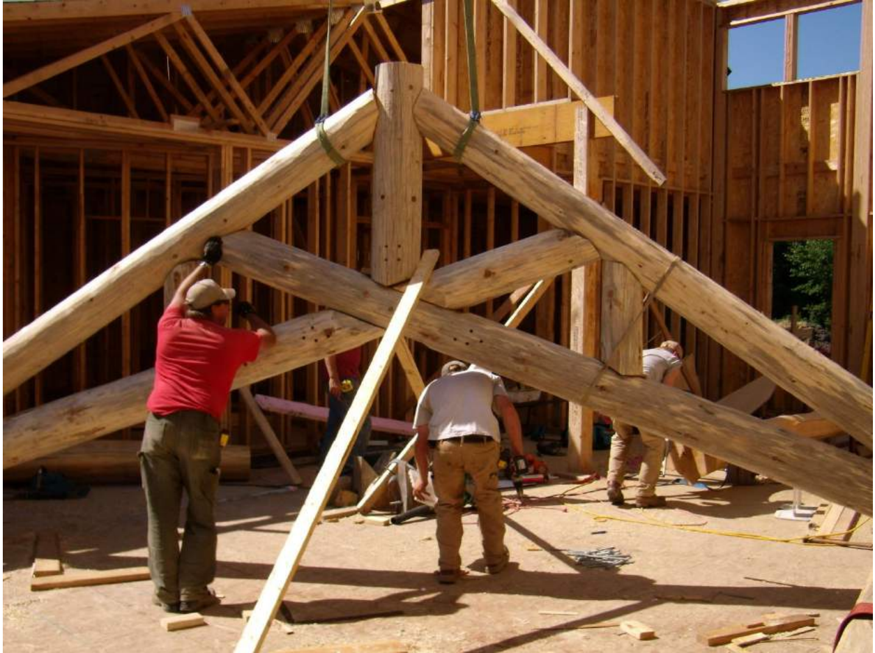
log scissor truss
