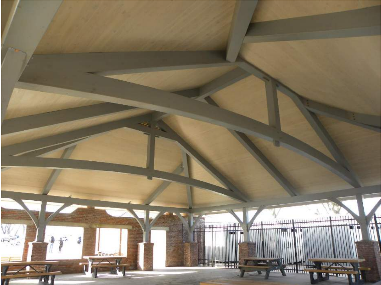
CLT panels over glulam trusses with traditional joinery
