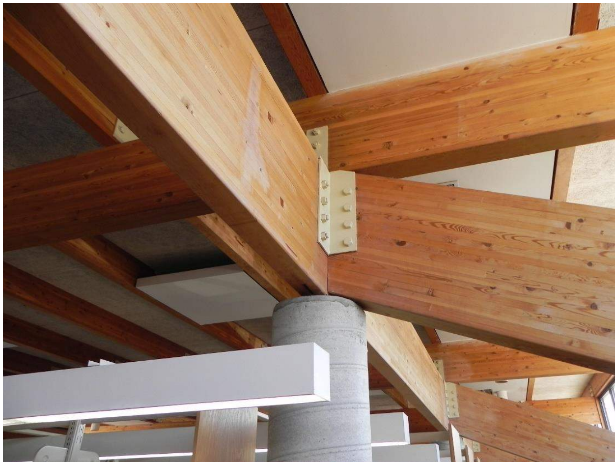
Traditional style glulam connection
