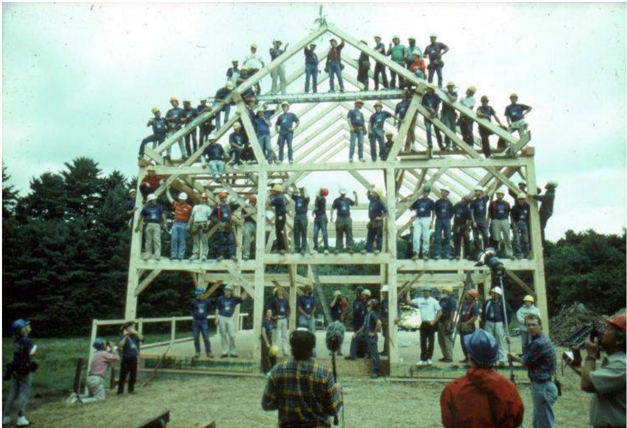
Barn frame topped out on This Old House photo credit – Steve Thomas
