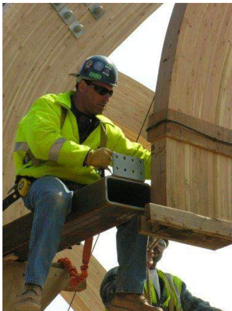
Ironworkers on high timber
