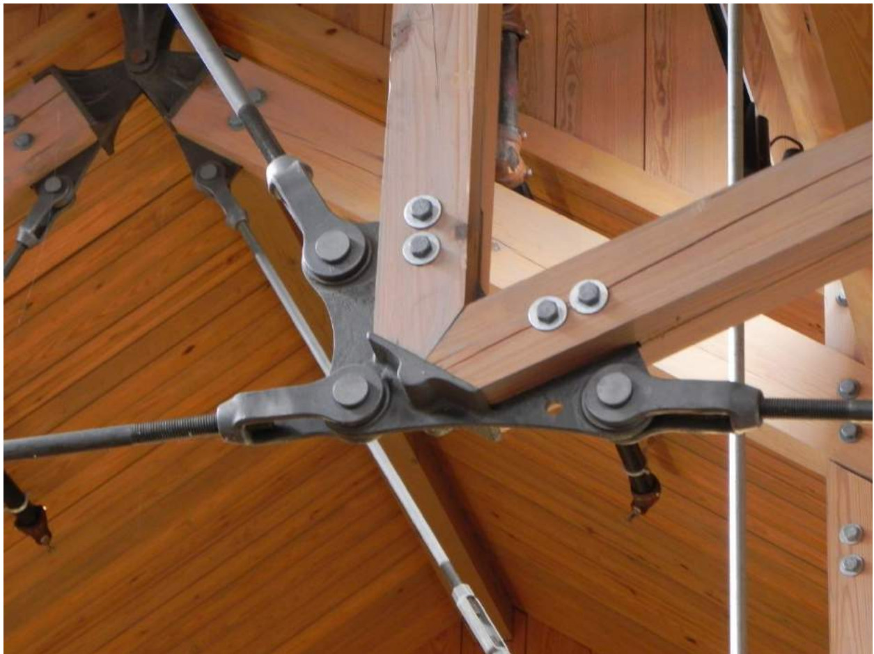
Cast steel connection hardware
