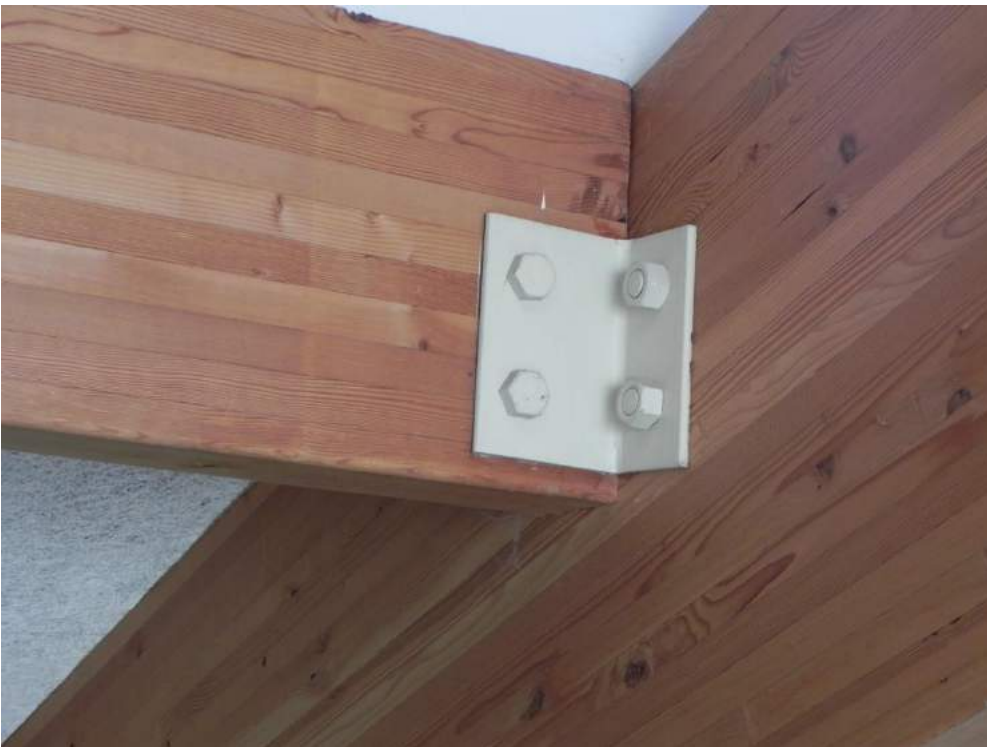
Glulam timber connections often emulate structural steel connections
