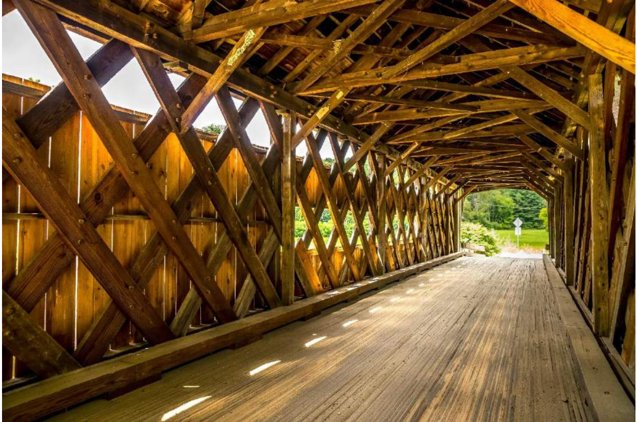
Worrall Bridge, Rockingham, Vermont; photo credit - Alamy
