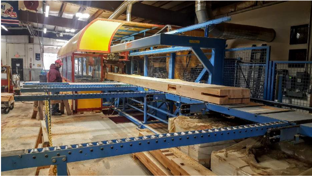
The Hundegger in action; photo credit – South County Post & Beam
