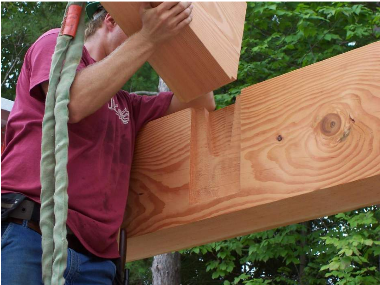
Rounded dovetail joints are easy with a Hundegger
