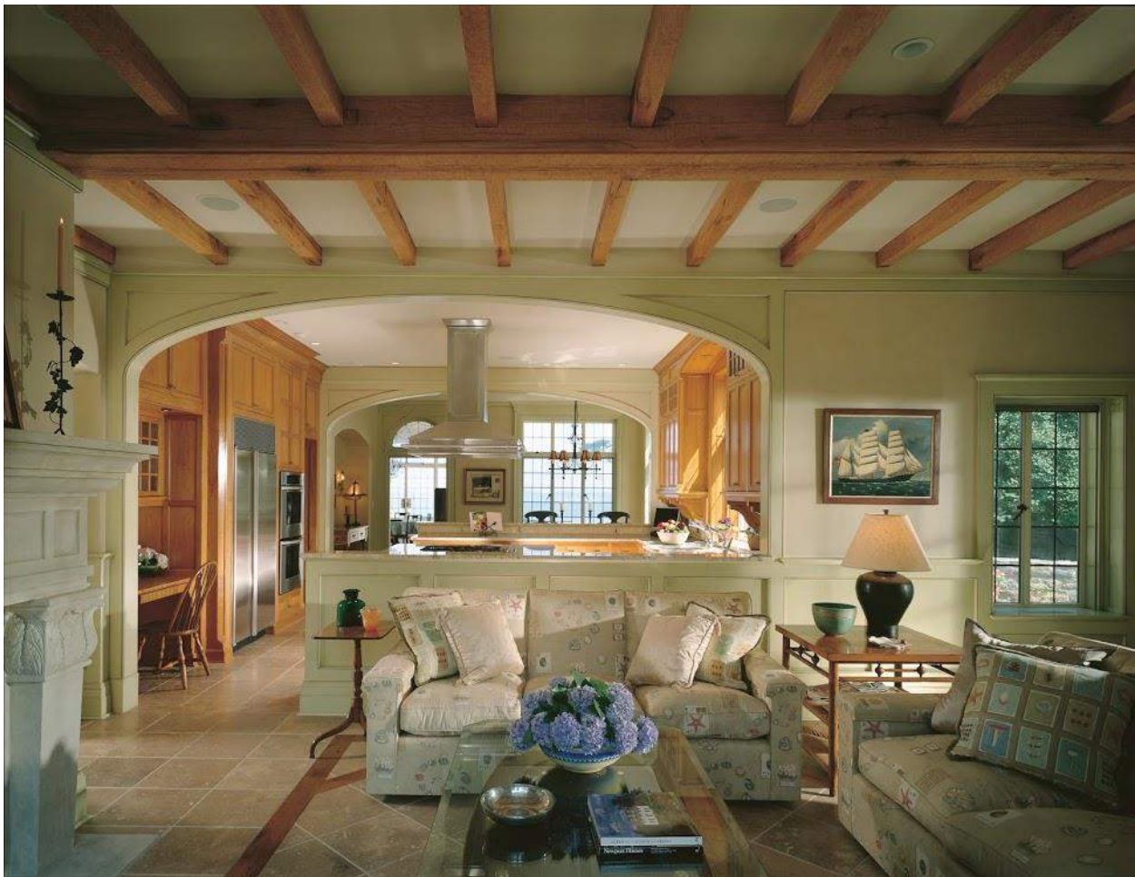
A great room ceiling with reclaimed white oak trimber summer beam and joists photo credit – E.M. Rose Builders
