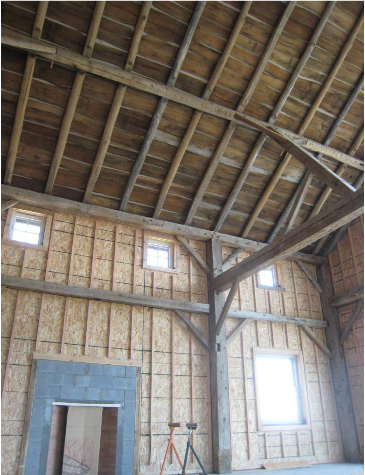
SIP panels enclose and support a restored barn frame
